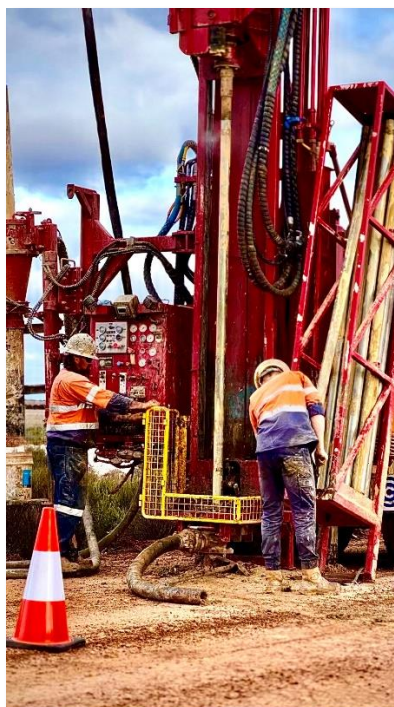
Figure 1: AC Rig on site
